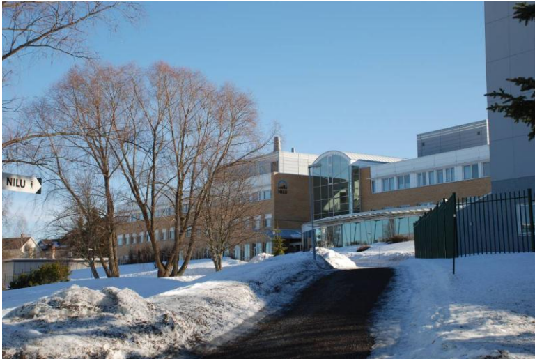
Very modern building of NILU in Kjeller.
