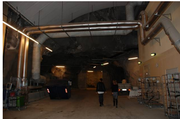
Large space for depositories.
